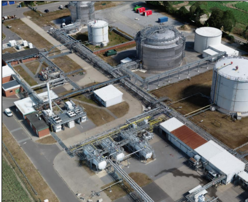
Figure 10: Interactive, textured 3D model of a gas facility, created from images taken by a DJI Phantom 4 RTK; Agisoft Metashape photogrammetry software (Haske 2021).
