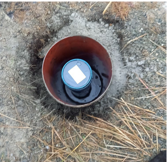
Figure 7: The drilling work for a piezometer in Siersza. [3] [5]
